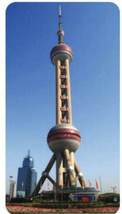
▲ The Oriental Pearl Tower in Shanghai is over half a kilometre high. In high winds, its top can move by a quarter of a metre. But, being elastic, its steel and concrete structure always returns to its original shape.
