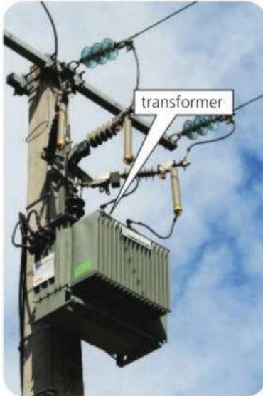
▲ A transformer connected to local power lines
