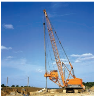
▲ Figure 5.10 When the mass falls, it gains kinetic energy and drives the pile into the ground.
