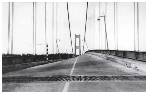
▲ Figure 17.18 The Tacoma Narrows bridge disaster
