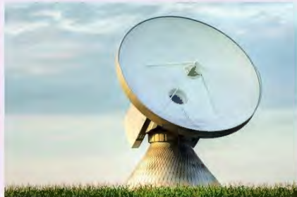
▲ Figure 10.16 Radio telescopes have concave reflecting dishes so that the signals from space reflect and converge onto a detector that is placed in front of the dish.
