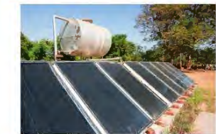
▲ Figure 17.14 Solar heating panels used to heat water
