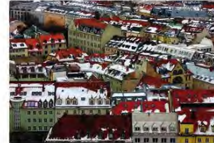
▲ Figure 15.17 Loft insulation makes a big difference to heat loss through the roof.
