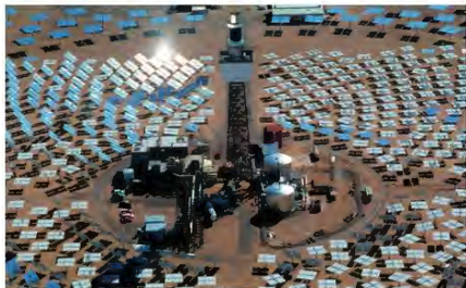
▲ Figure 17.16 A large number of mirrors focus heat from the Sun on a boiler in the tower at the centre. The steam produced drives a turbine to generate electricity.
